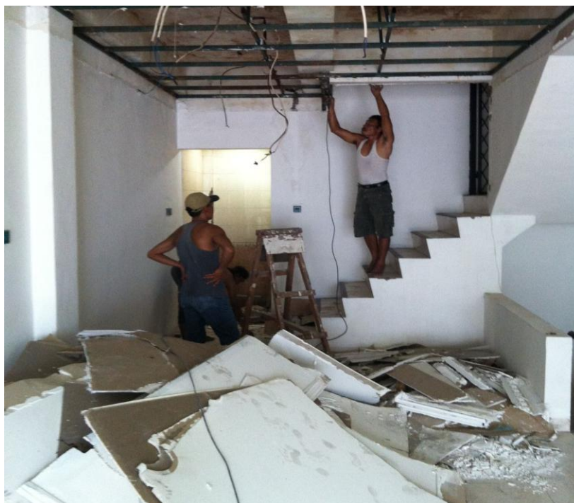
Early stage of clinic renovation.
